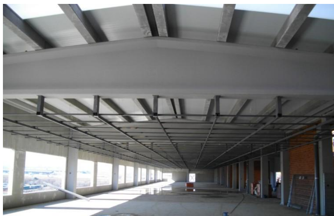
Figure 1: Reinforced concrete rafters.
