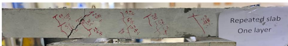
Figure 5: Cracks Pattern for Bottom and side Projections of Specimen (BR1.2), under repeated load test.
